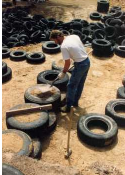
Figure 2: Image of a partially built tire wall and the construction process
