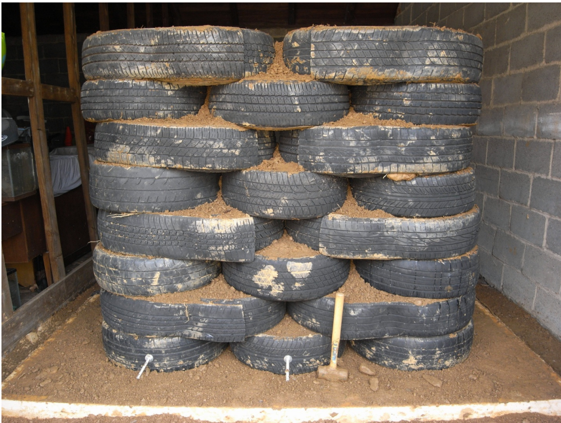
Figure 12: Constructed small-scale wall with no lateral support
