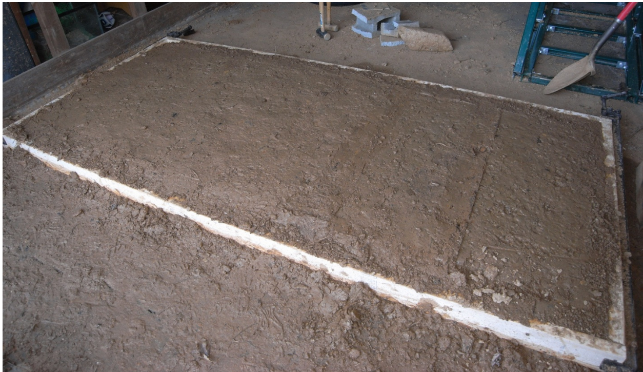
Figure 6: Wooden Frame foundation filled with compacted soil used for all friction and wall tests
